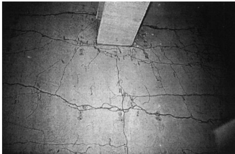
Fig. 25. Photograph of the top surface of the concrete slab at the joint after testing [26].
