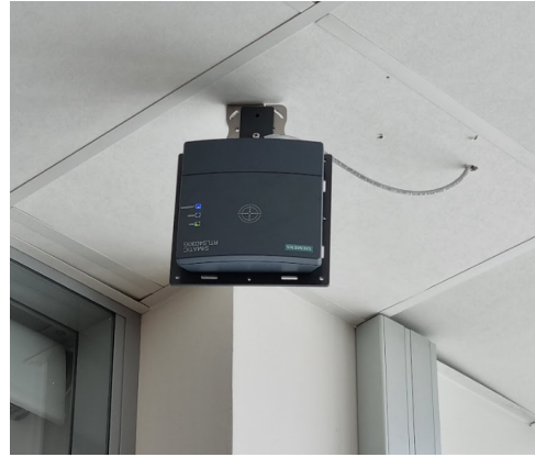
(b) : Vertical mounting of the gate
