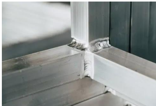
Figure 17: Picture of three profiles permanently connected with welding
