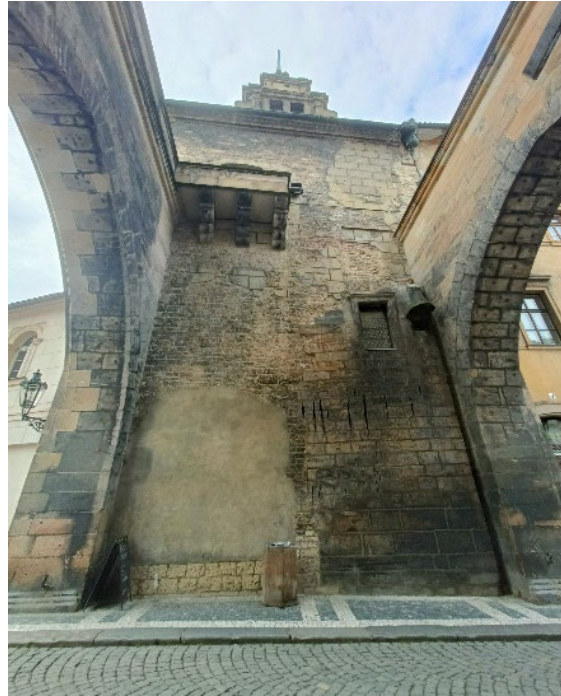
Figure 3.3 The connection between the Tower and the gate – North Façade
