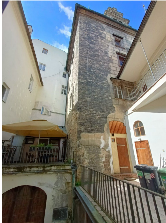
Figure 2.6 Eastern Façade – The accessible to the via a gallery in the northern wing of the house.
