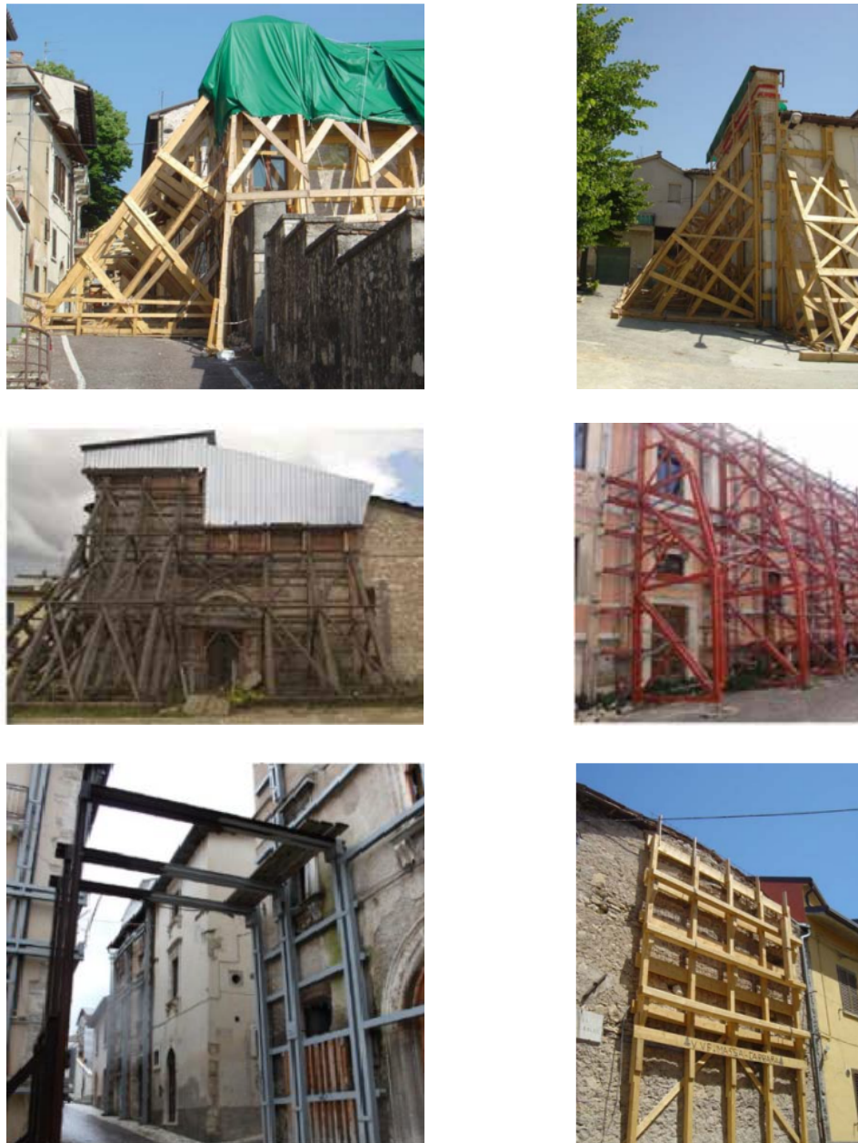
Fig 1 : temporal shoring timber structures stabilizing damaged masonry structures
