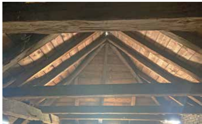
Fig 53: First section of timber roof, facing north
