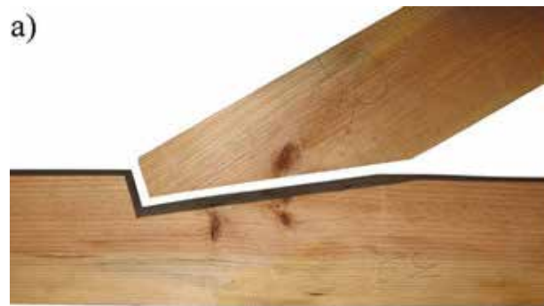
Fig 65 : Simple front notched connection without metal parts
