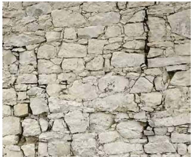
Fig 25: 1x1 square of opuka masonry wall
