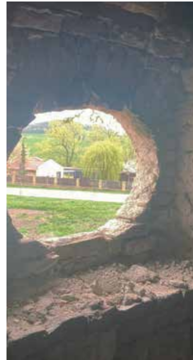
Fig 41: Circular opening from interior
