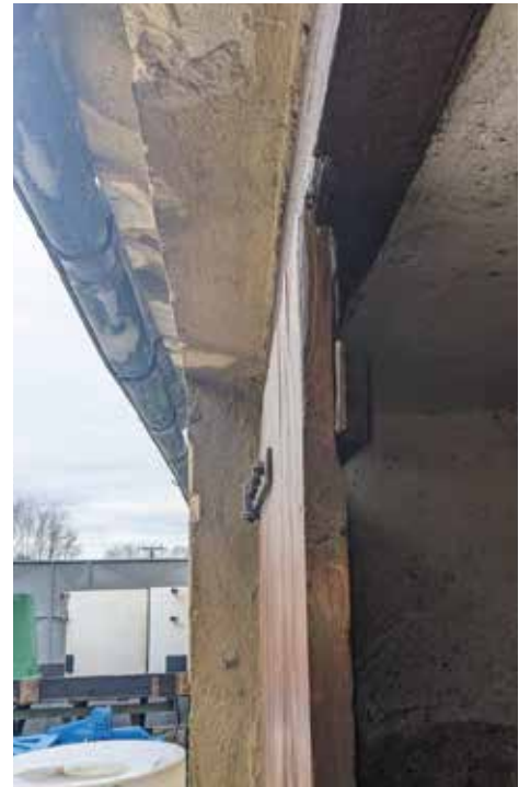
Fig 46: Different color & texture interior and exterior plaster renders
