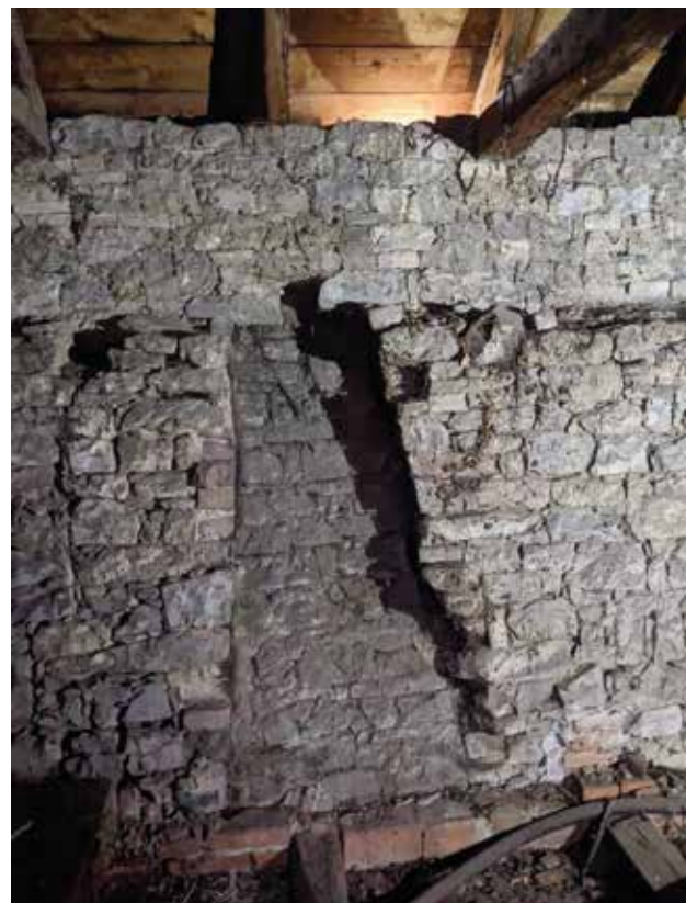
Fig 48: Former chimney shaft
