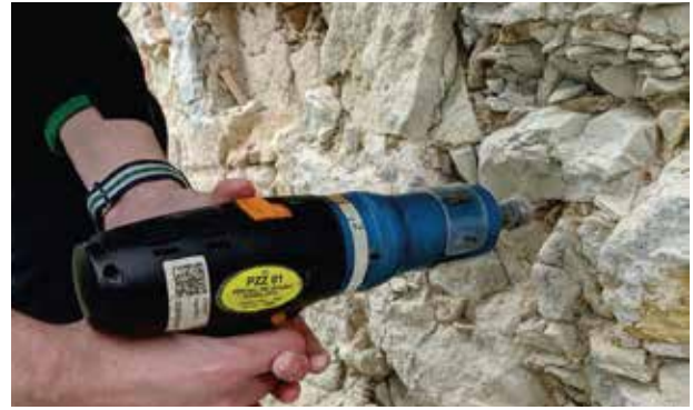
Fig 27: Drilling in joints for mortar samples
