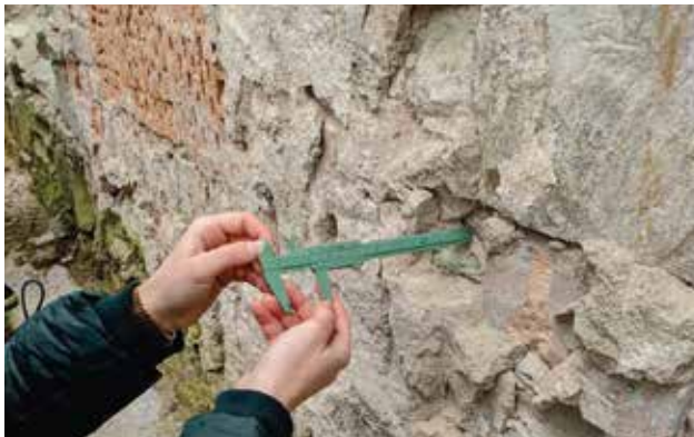
Fig 28; Borehole depth measurement
