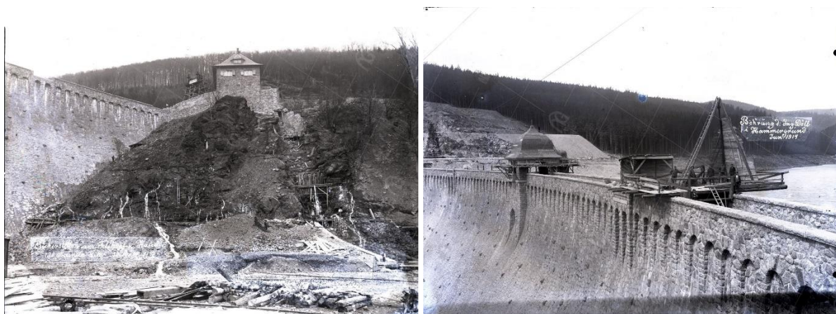
Figure 2.7 - First sealing work (a) Seepage in the left bank impoundment appeared soon after the first filling of the reservoir, March 25, 1914; (b) Additional sealing work in the left slope, June 1914, © Panoráma starého Mostecká.
