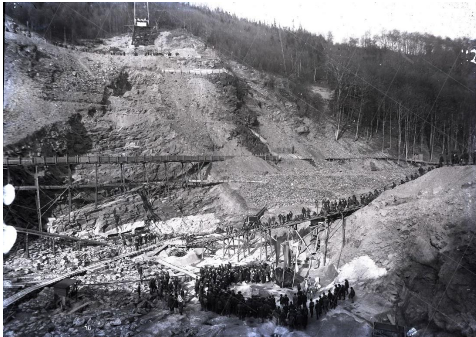
Figure 2.3 - Picture of the ceremonial laying of the foundation stone, 4 May 1912, © Panoráma starého Mostecka.
