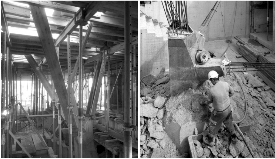
Figure 9.8: Illustration of RWPA inspirational column (see Figure 2.12) construction process
