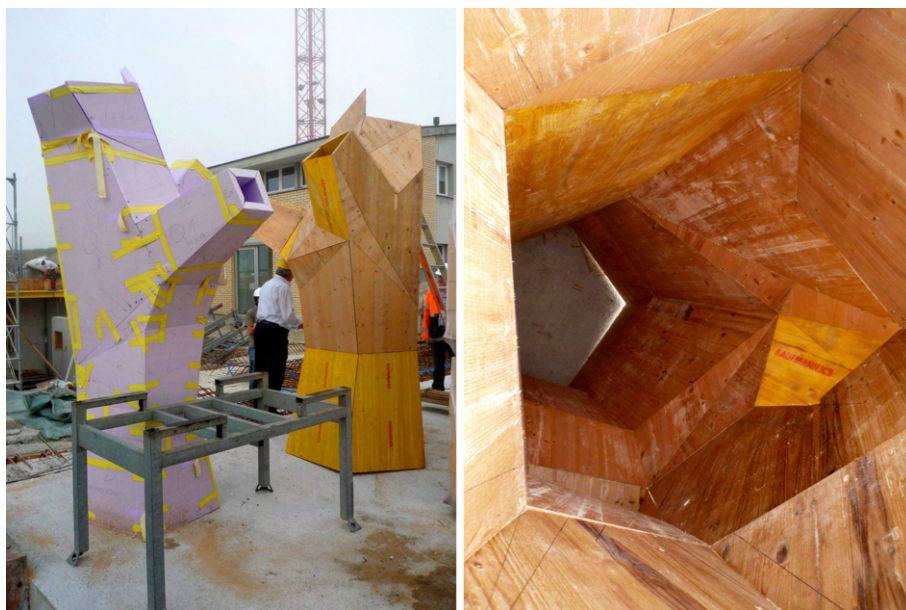
Figure 9.7: Illustration of RWPA inspirational column (see Figure 2.12) formwork
