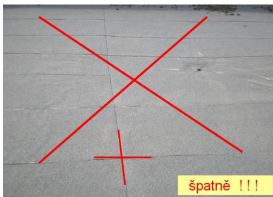
Obr. 7 – Absence T – spoje u asf. izolace [16]
