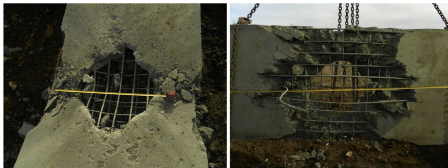
Fig. 19. Damage to reference specimen No. 1 after the blast. Top view (left image), bottom view (right image).
