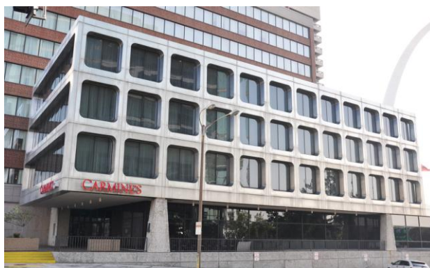
Obr. 1.7 - The American Zinc Building, St. Louis, Missouri [5]
