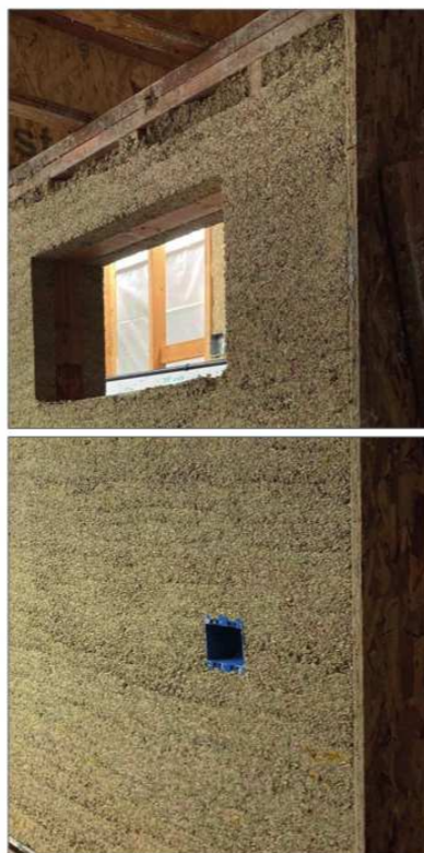
Poured in place Hempcrete wall.
