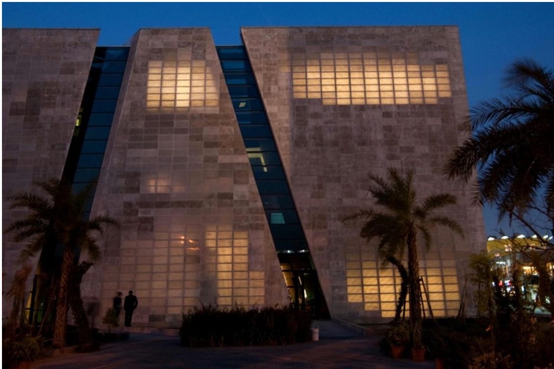
Figure 16: Italy EXPO Pavilion, Shanghai, China, 2010 [28]
