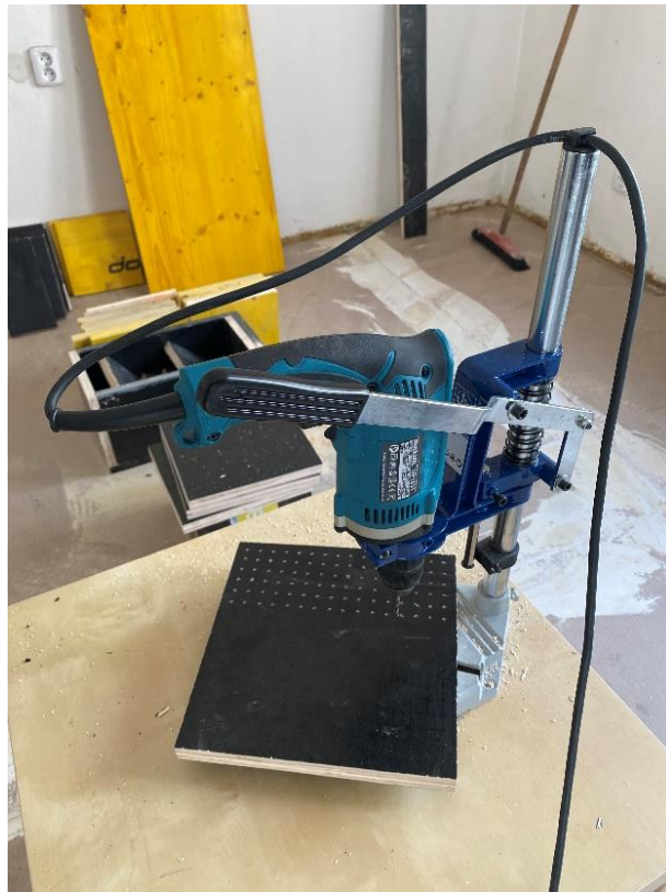
Figure 52: Making penetrations for optical fibers
