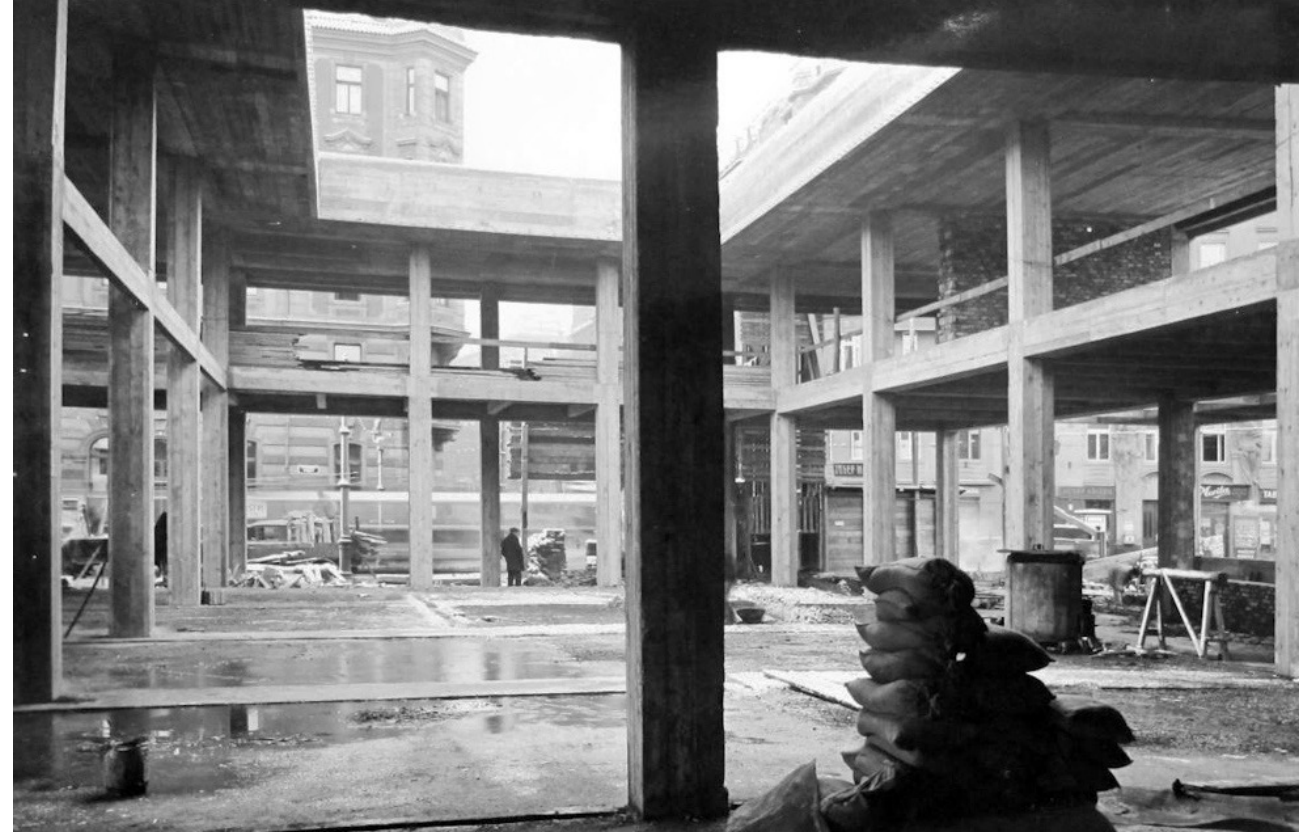
158. under construction, 1929. photo: ncvu archive
