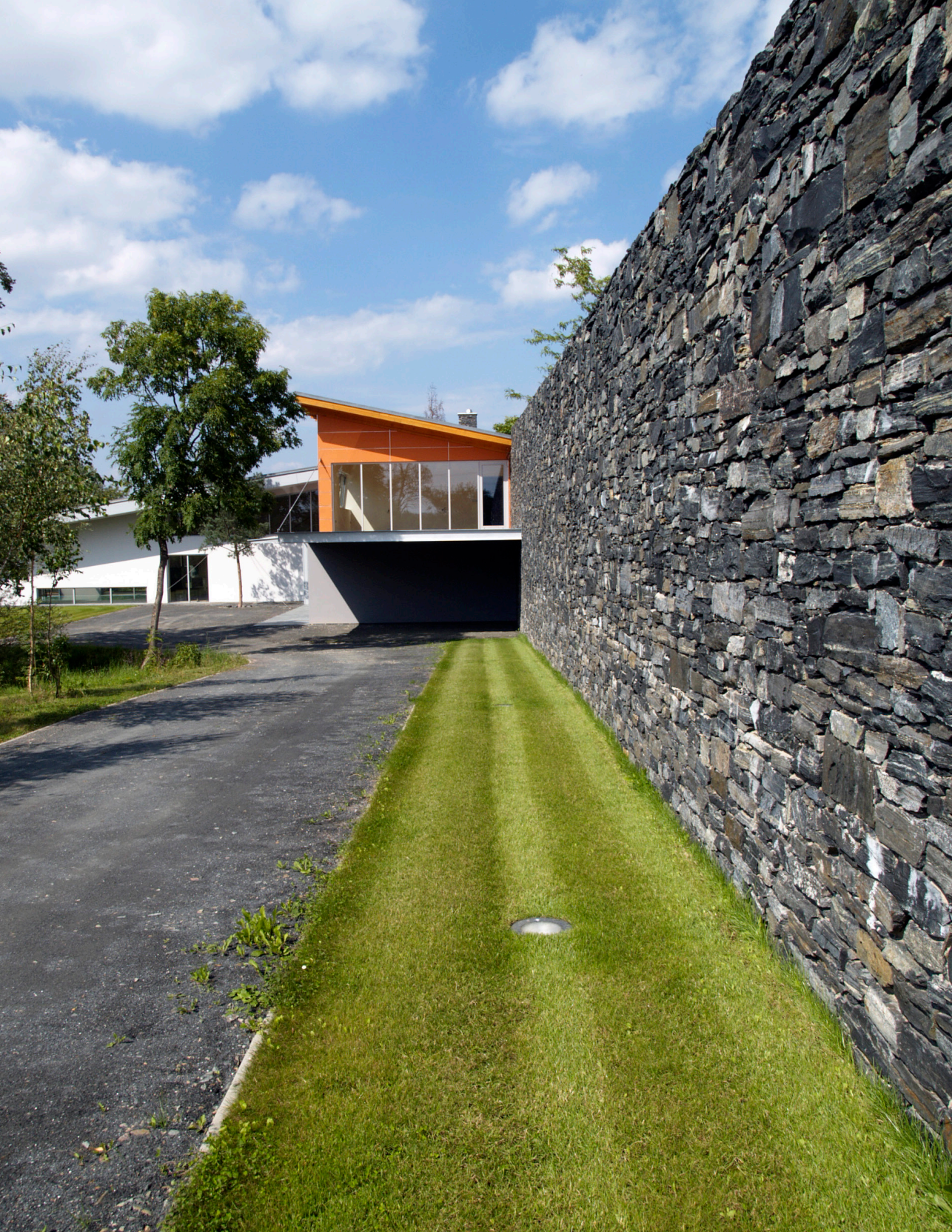
104. movement along stone wall photos: radim jareš
