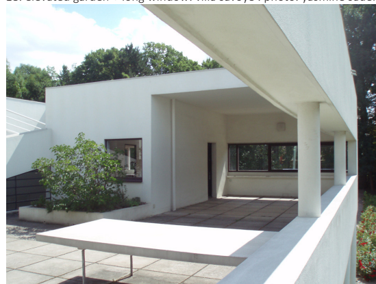
18. elevated garden + long window: villa savoye . photo: yasmine sadek
