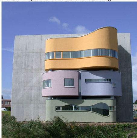
83. frontality, wall house 2. photo: liao yusheng
