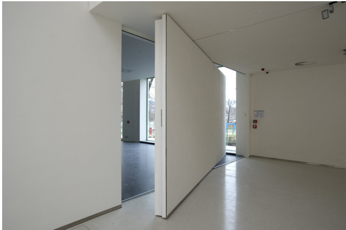
177. new pivot door linking main gallery to cafe/bar. photo: hmarchitekti
