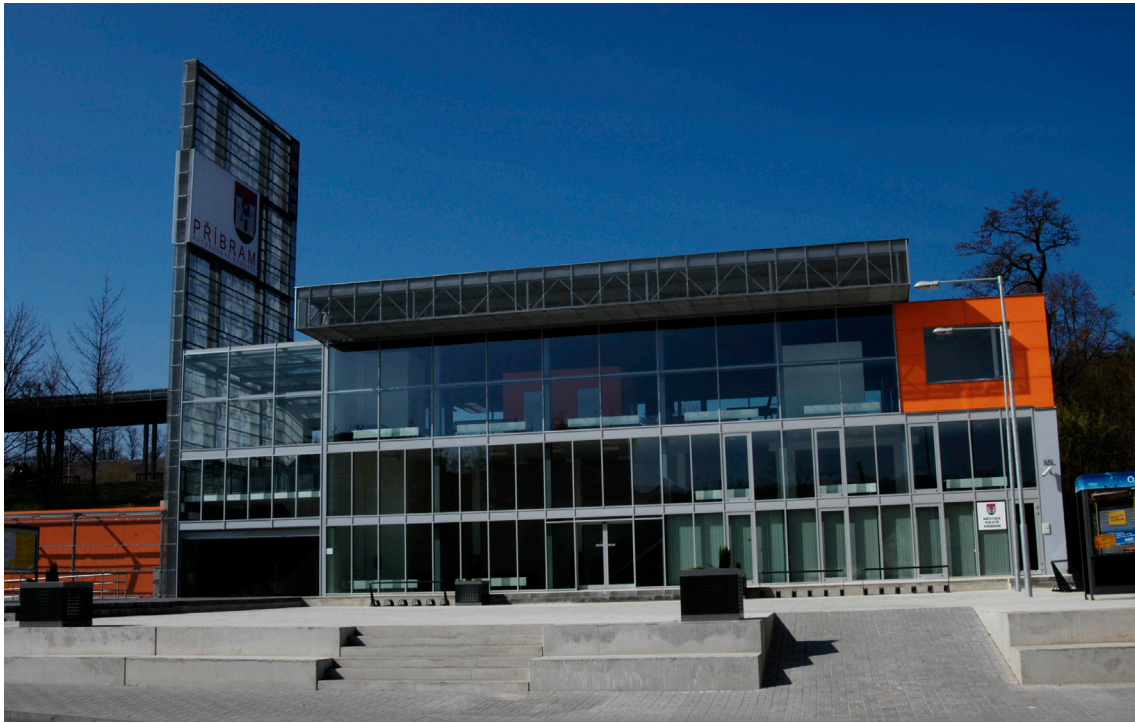
149. lower square. photo: hmarchitekti
