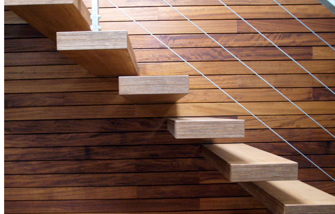
138. cantilevered step. photo: radim jareš
