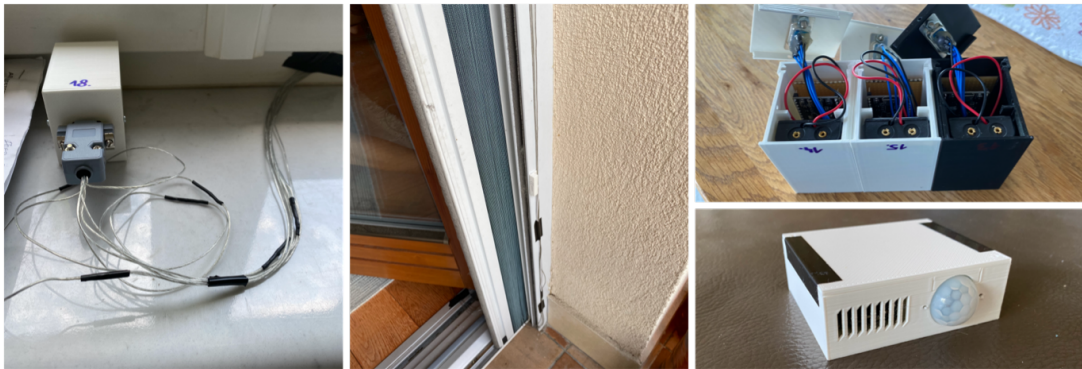
FIGURE 2. Monitoring sensors in the apartment (window opening, shading, motion detection).
