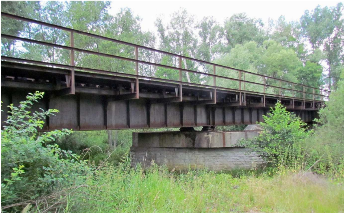
Figure 4.3: Bridge B2 – plate girder bridge without bridge deck.
