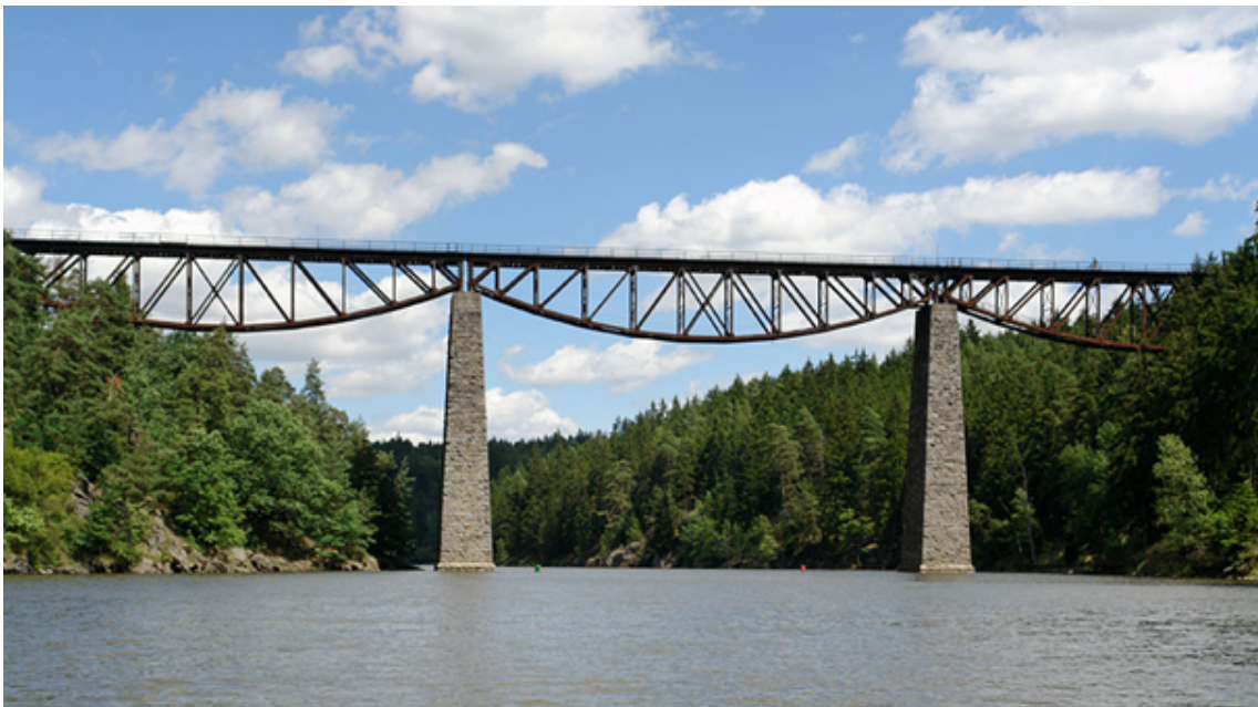
Figure 4.11: Bridge B6 – truss girder bridge with upper bridge deck.
