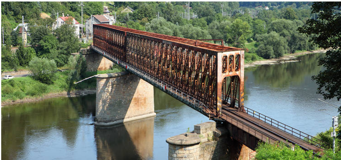
Figure 4.14: Bridge B8 – truss girder bridge with lower bridge deck.
