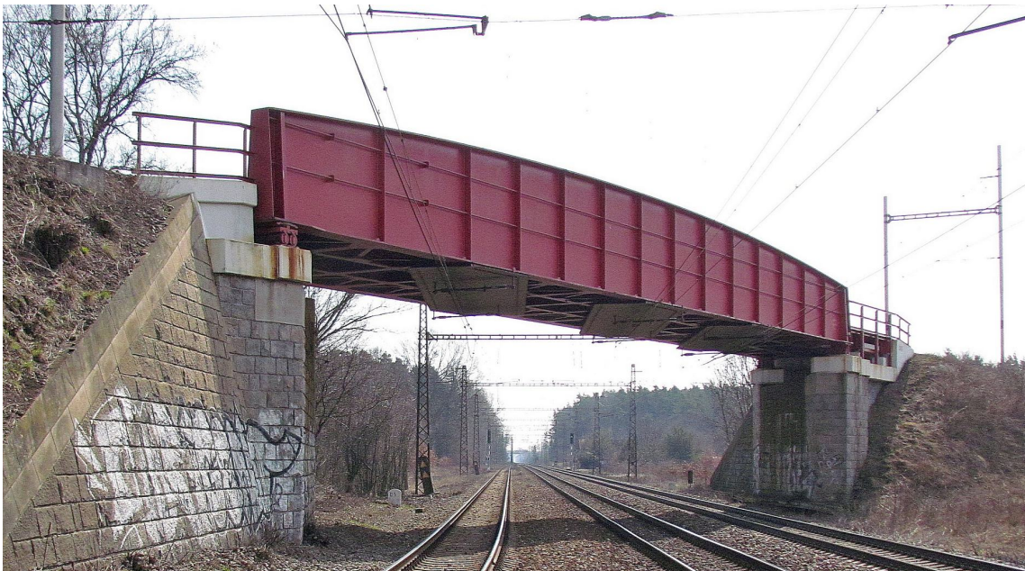
Figure 4.7: Bridge B4 – plate girder bridge with lower bridge deck.
