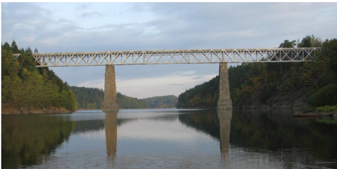
Figure 4.12: Bridge B7 – truss girder bridge with intermediate bridge deck.
