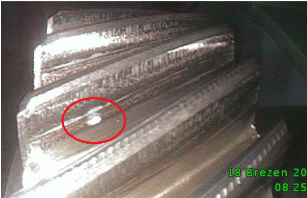
Figure 7-23: Pitting on PM HIP:ed gearwheel (6 th speed) – gearset 2 - after 41 hours
