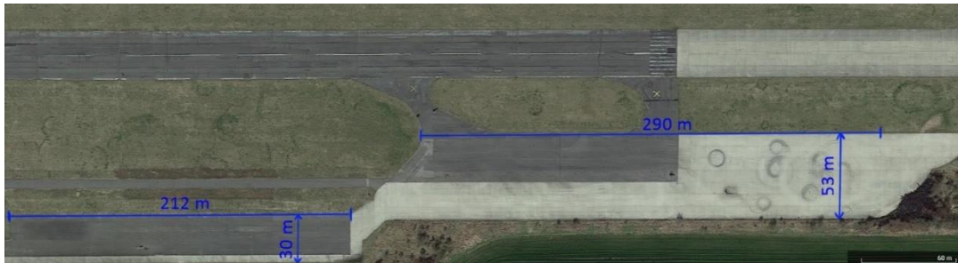
Figure D 5 - LKPC-27 taxiway and apron tarmac area
