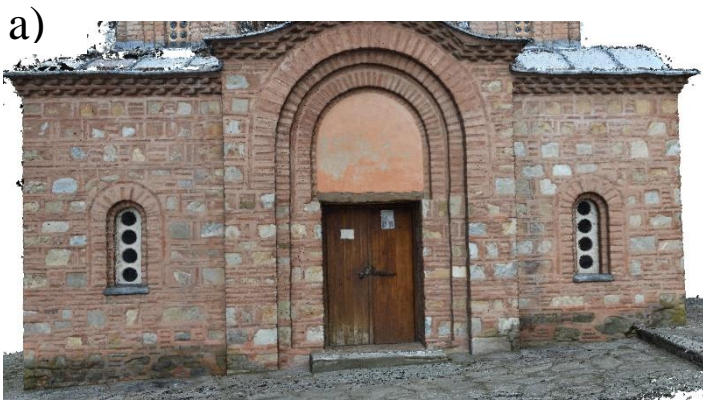
figure 7 - Textured point cloud from Close-range photogrammetry - details
