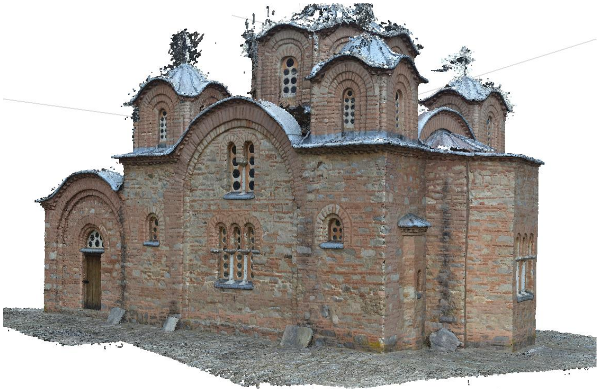
figure 8 - Textured point cloud from Close-range photogrammetry – north-east view
