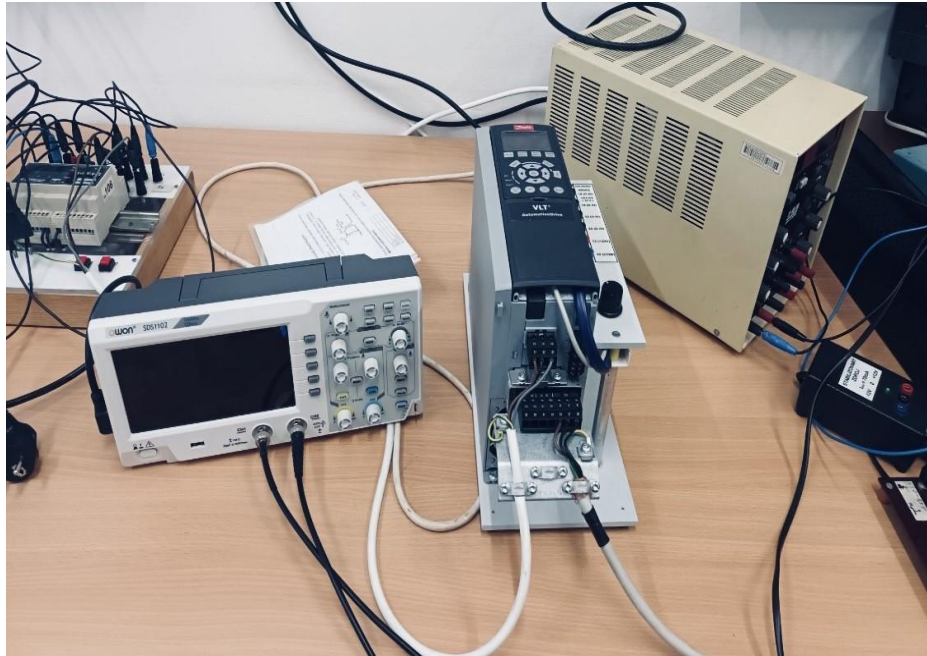
Figure 13: Connection of oscilloscope and wattmeter to HVAC VLT Drive
