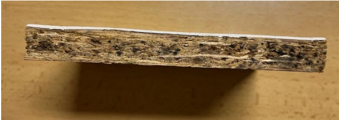
Figure 26: OSB with plaster coating with visible delamination.
