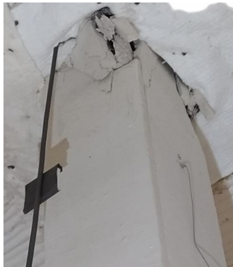
Figure 26: Detail of local failure at the edge of the test specimen with Knauf Vermiplaster
