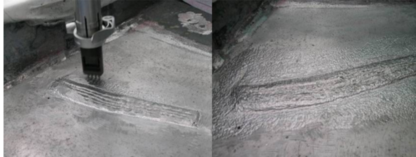
Figure 1.20: Application of ultrasonic peening technology to localized AA5456-H116 aluminum crack repair [93].
