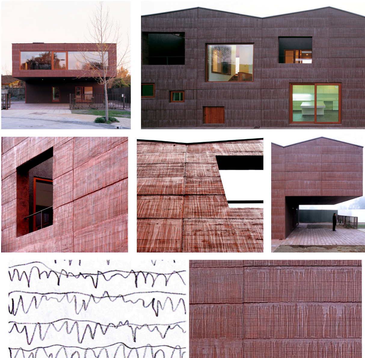
▽ Obr. 76 Detaily fasády [64]
