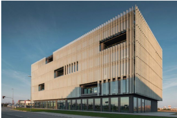
Figure 4.78 Office Building Konplan (source: Petr Polák, archiweb.cz)
