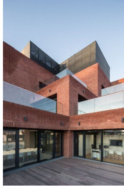
Figure 4.85 Prague 7 Townhall roof (source: Tomáš Slavík, archiweb.cz)
