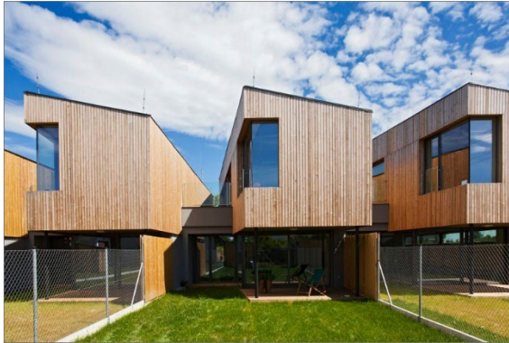
Figure 4.20 Terraced Houses Zruč (source: Jana Labuťová, archiweb.cz)
