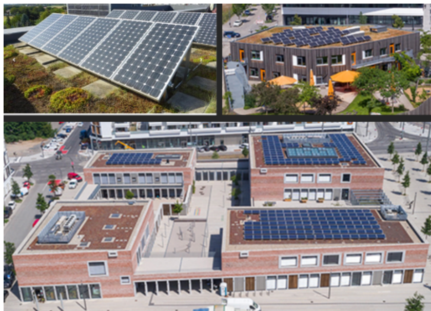
Figure 3.3.9 Photovoltaic solar panels arrays (source: City of Heidelberg, 2022)
