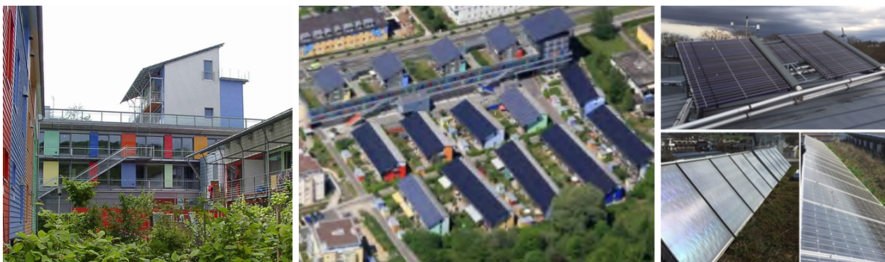
Figure 3.1.6 Plus-energy residential complex (left and middle) (source: (City of Freiburg, 2008) ); Solar thermal (top right) and Solar Photovoltaic (PV) (bottom right) (source: Bardhyl Rama).
