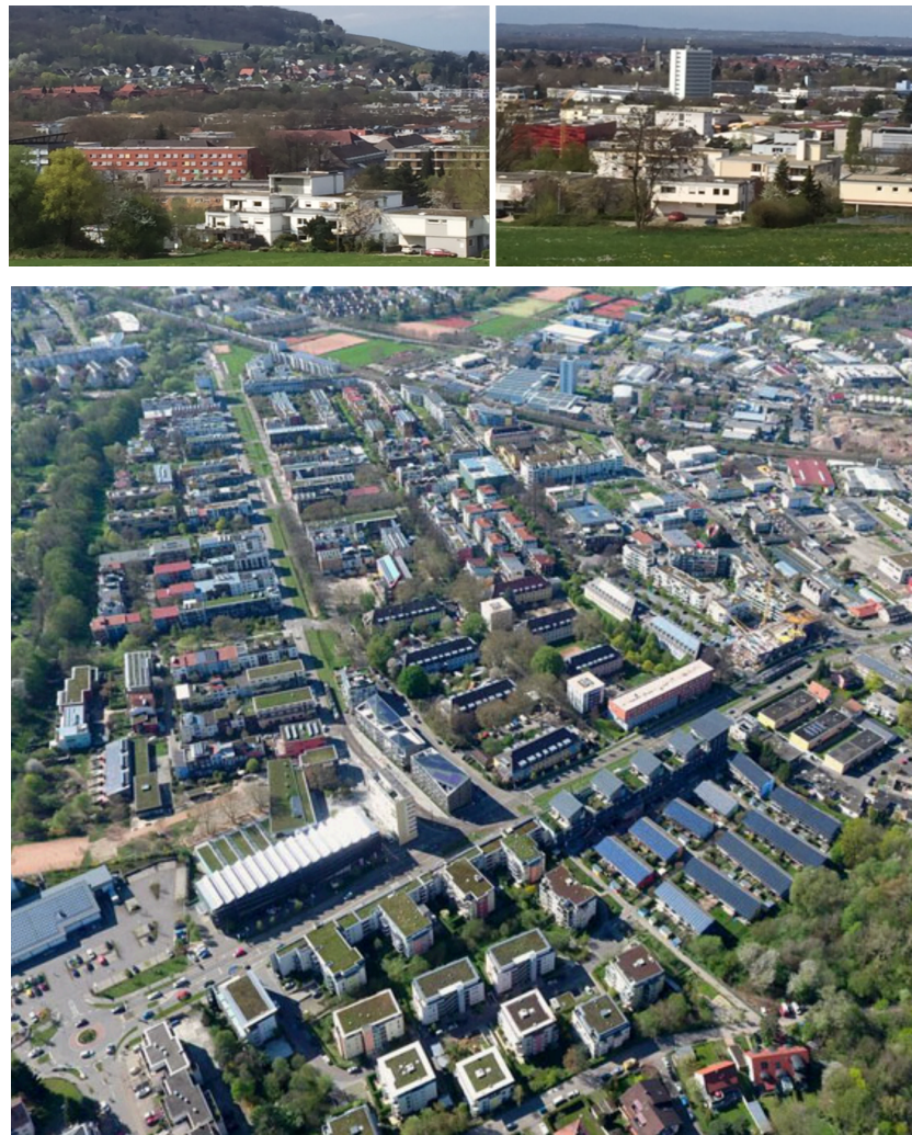
Figure 3.1.2 The view from the nearby hills (top) (source: Bardhyl Rama), and the aerial photo of Vauban district (bottom) (source: City of Freiburg, 2008).
