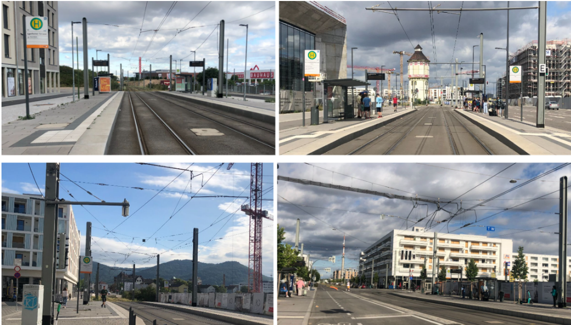
Figure 3.3.12 View of the tram line stops (source: Bardhyl Rama)
