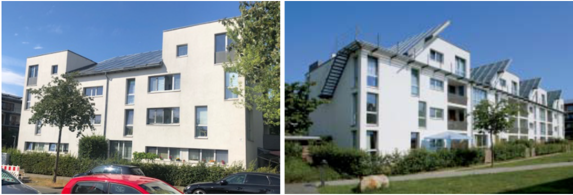
Figure 3.2.7 View of Solarcity building (source: Bardhyl Rama (left), (Rumming et al., 2004b) (right))
