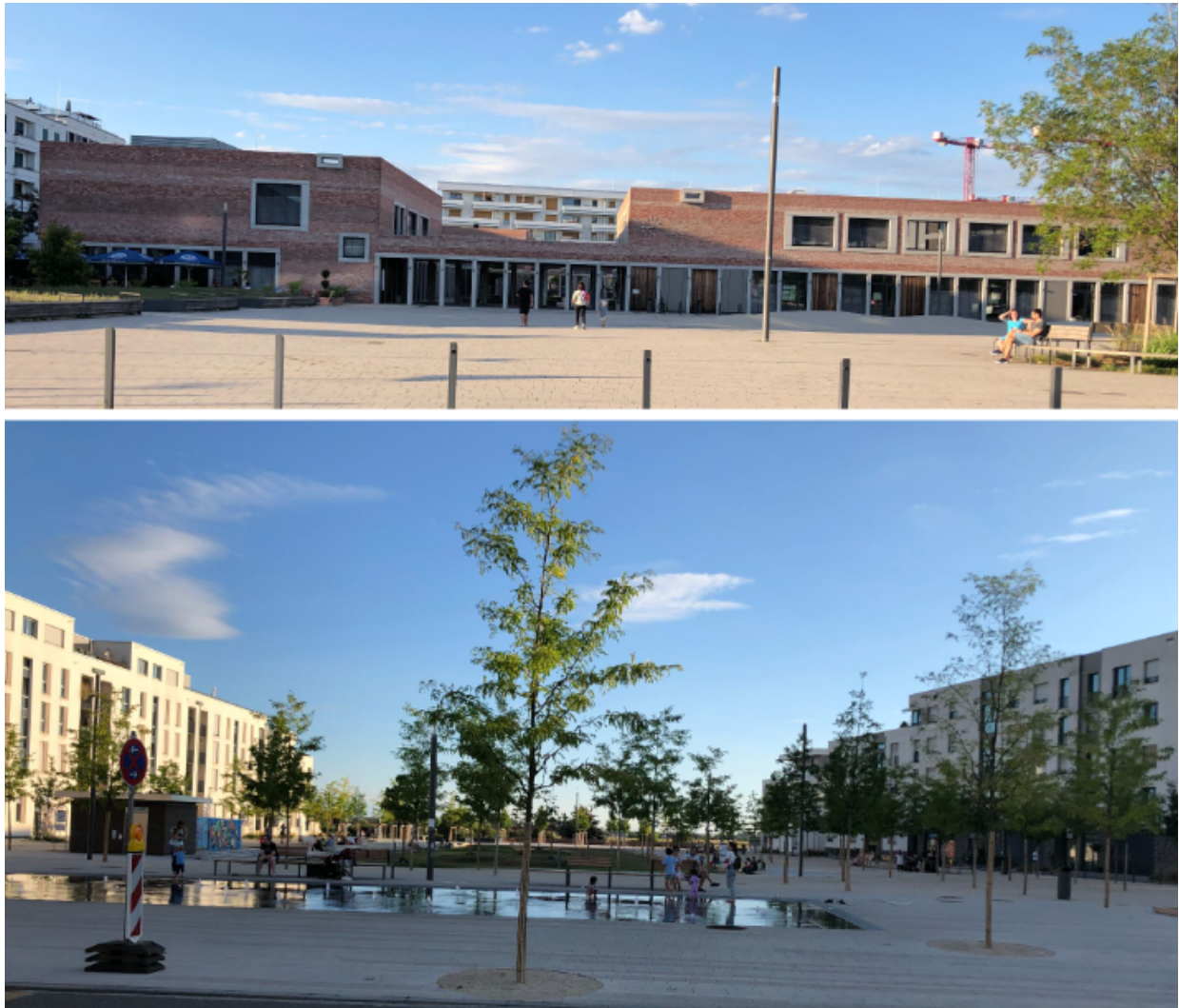
Figure 3.3.15 Gadamerplatz and the B 3 center (top) and Pfaffengrunder Terrasse (bottom) (source: Bardhyl Rama)
