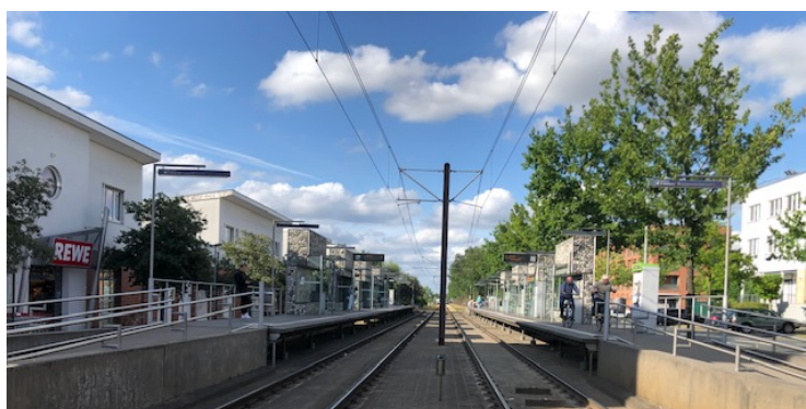
Figure 3.2.13 View of one of the main Kronsberg tram stop (source: Bardhyl Rama)
