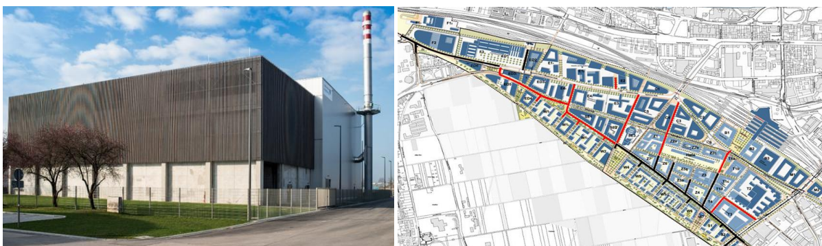
Figure 3.3.10 Combined Heat and Power (CHP) wood-fired thermal power station (left), district heating network (right) (source: City of Heidelberg)
