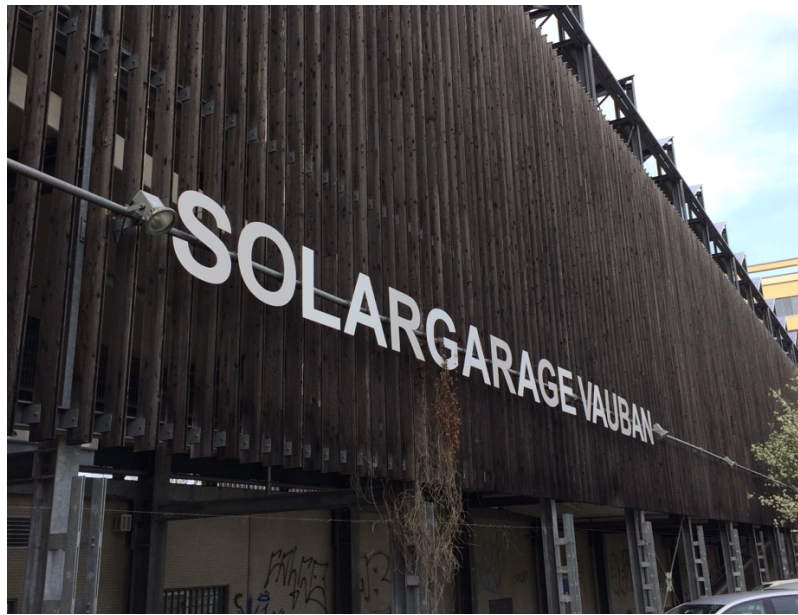
Figure 3.1.11 District parking garage (source: Bardhyl Rama)
