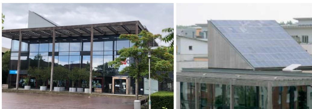
Figure 3.2.11 Photovoltaic installation at KroKuS (source: Bardhyl Rama (left), (Rumming et al., 2004b) (right))
