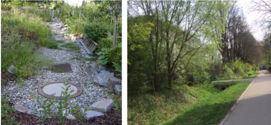
Figure 3.1.18 Rainwater collection, infiltration area (left) (source: (City of Freiburg, 2008) ); view of functioning open water collection/drainage ditch (source: Bardhyl Rama)
