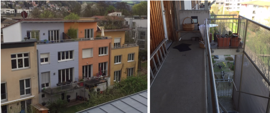
Figure 3.1.4 Group owner's four-story multi-family houses (left), access to upper unit via outside balcony (right) (source: Bardhyl Rama).
