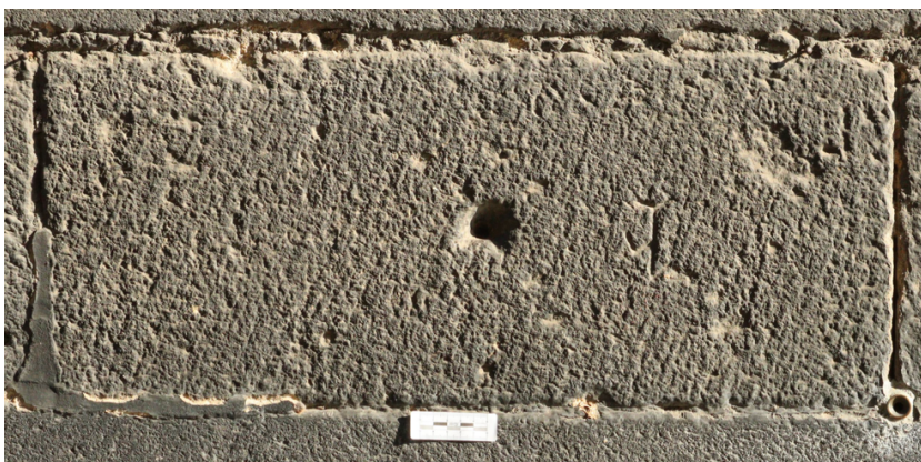
FIGURE 5. Malá Strana – Malostranská Bridge Tower, 2nd half of the 15th century. Final realignment of the face in an oblique grid in parallel rows with a straight-edged chisel (photo by M. Cihla, taken from [13]).
