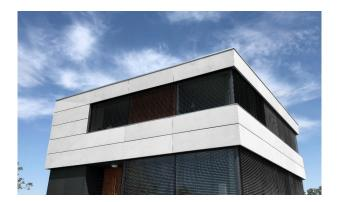
FIGURE 2. Carbon reinf. concrete façade white concrete - curtain wall.
