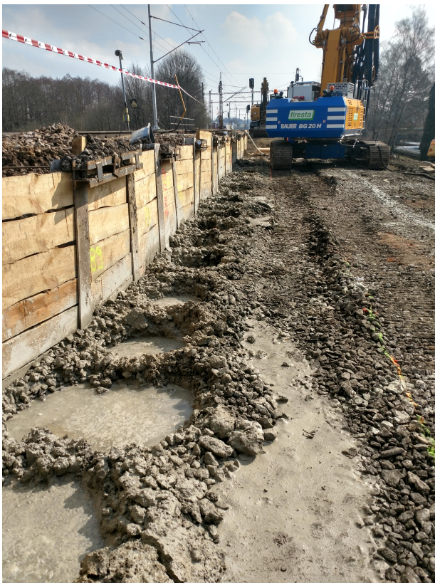
FIGURE 6. Construction of DSM columns at the Žďár nad Sázavou building site
