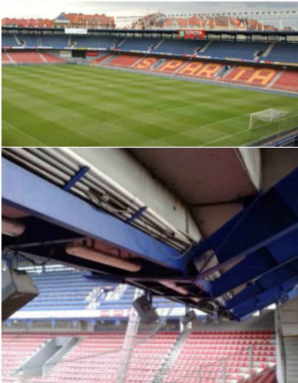
FIGURE 2. Platform construction: a) Letna Stadium – the overall view [8], b) Letna Stadium detail [1].
