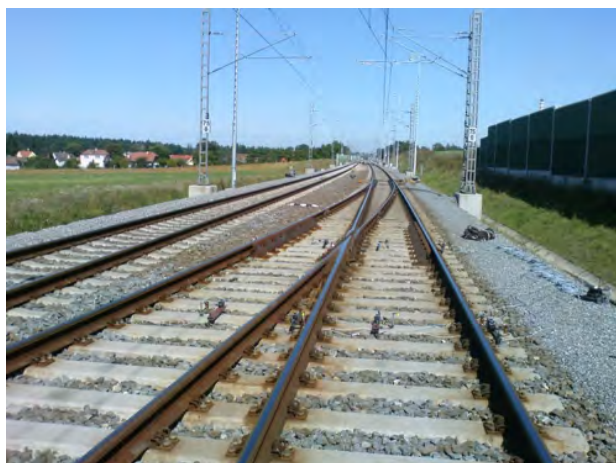
FIGURE 1. Test section in Plana nad Luznici railway station - under sleeper pads
