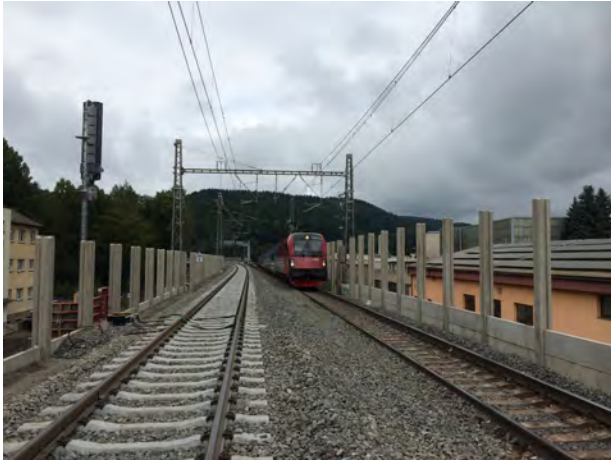
FIGURE 3. Installation of noise barriers in Usti nad Orlici
