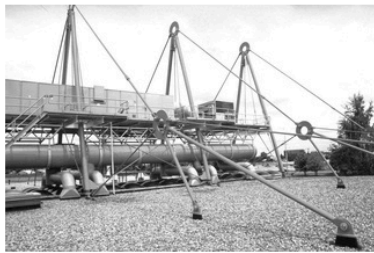
PAT Center - Structure
