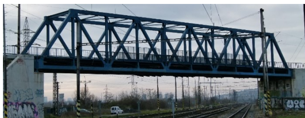
FIGURE 1. Steel truss railway bridge in Bratislava.
