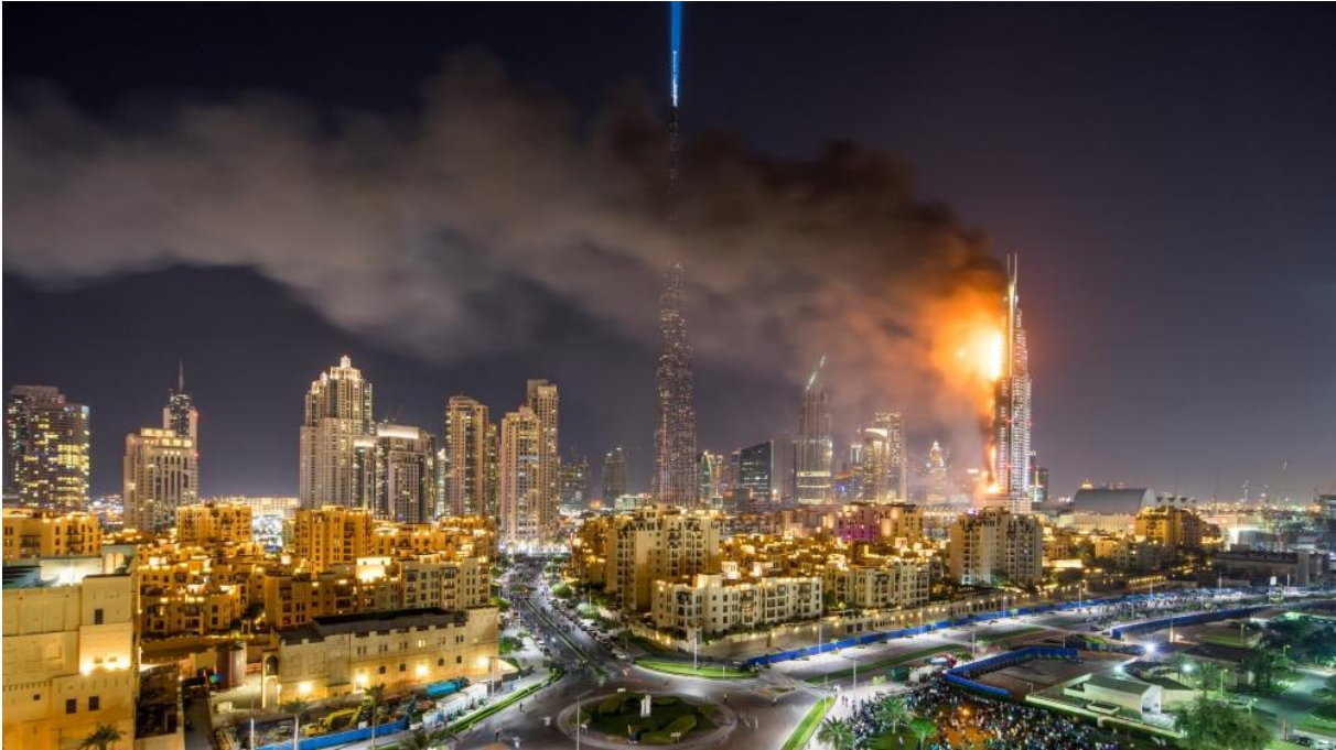
Fig. 1-8. Fire of Torch skyscraper, Dubai 2015[14].
