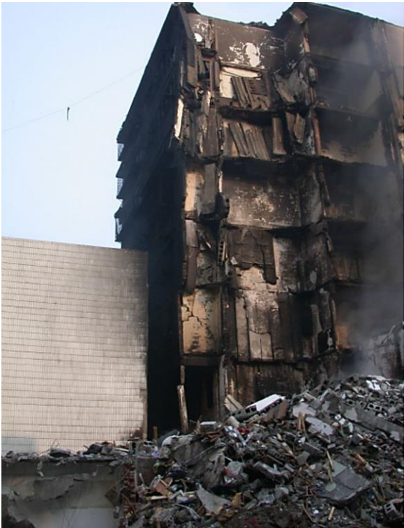
Fig. 1-6. Partial fire-induced collapse of Hengzhou building, China 2003 [13].
