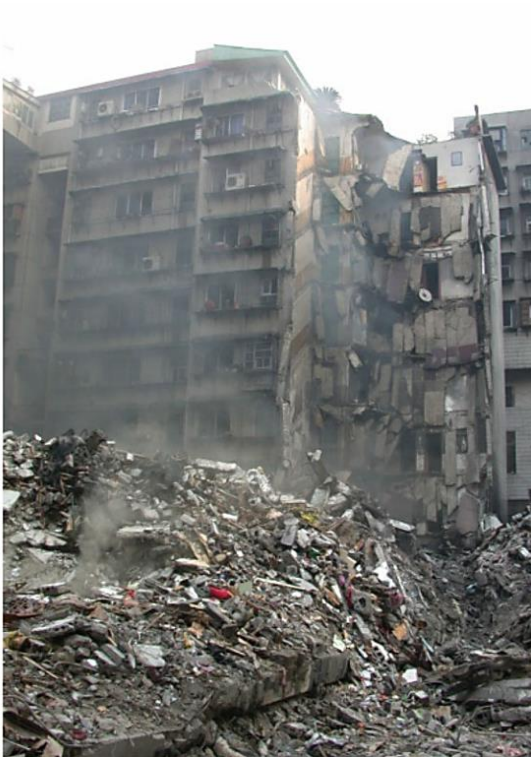
Fig. 1-6. Partial fire-induced collapse of Hengzhou building, China 2003 [13].
