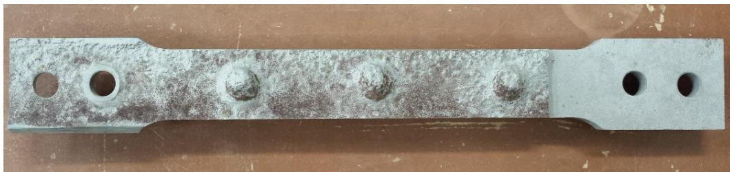
Fig. 38 Photo of tested specimen with a high level of corrosion (Example of a sample from group 3)
