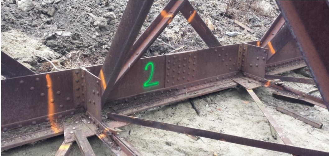
Fig. 26 Part 2 removed from the right-hand girder of the bridge structure
