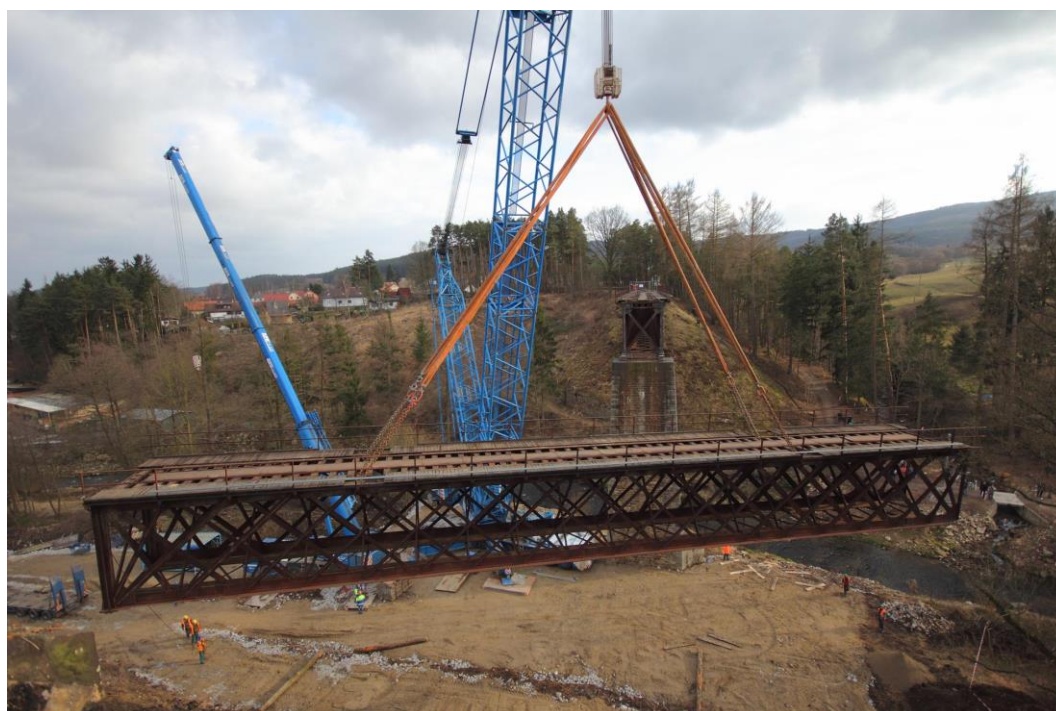
Fig. 23 Photo of Holubov Bridge during the reconstruction
