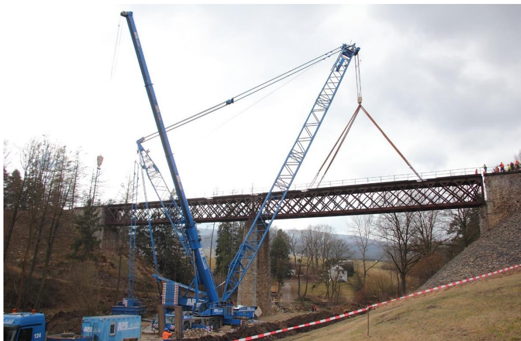
Fig. 22 Photo of Holubov Bridge during the reconstruction
