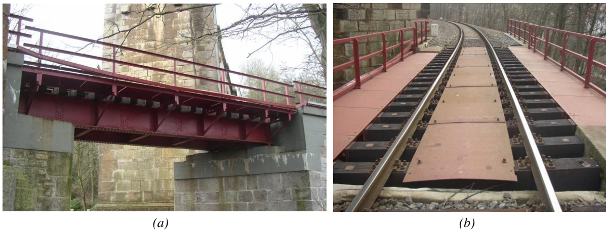
Fig. 91 Railway bridge: a) longitudinal view; b) view on the superstructure
