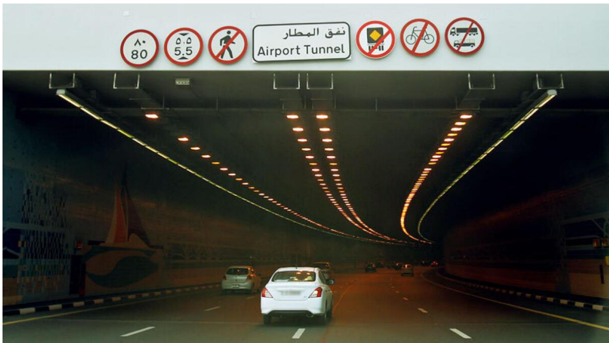
Obrázek 9: Vjezd do tunelu DIA [18]
