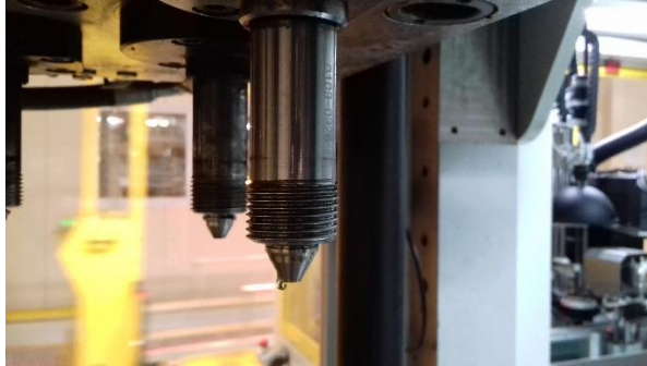
Figure 21 : Glycol leakage from the nozzle
