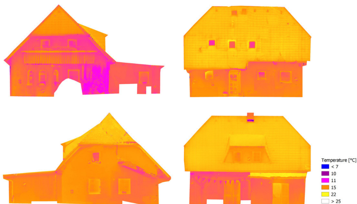
Figure 10. The resulting orthophotos augmented by thermal information.
