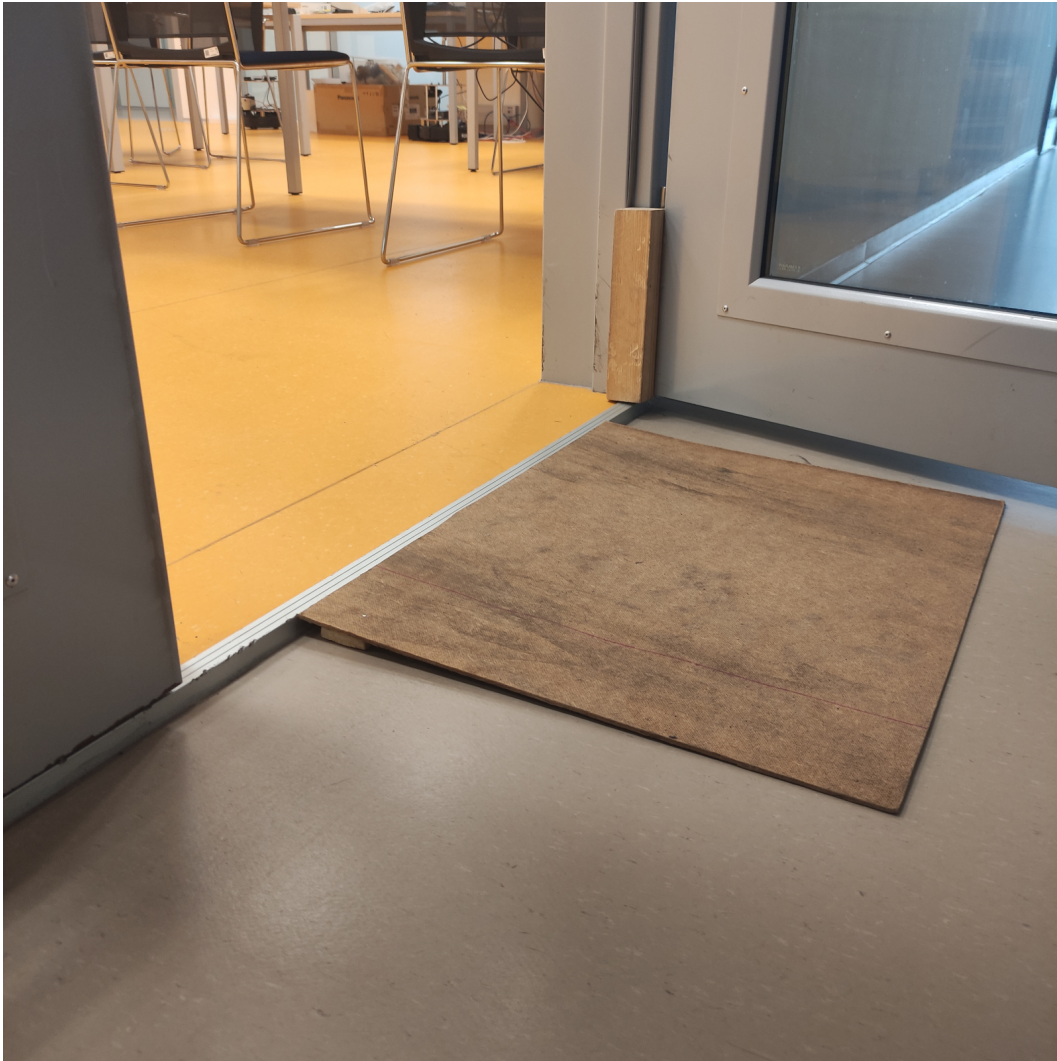
Figure 6.1. Ramp to move TIAGo over small steps.
