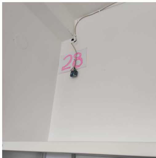
Figure 5.4: Installation of beacon 28
