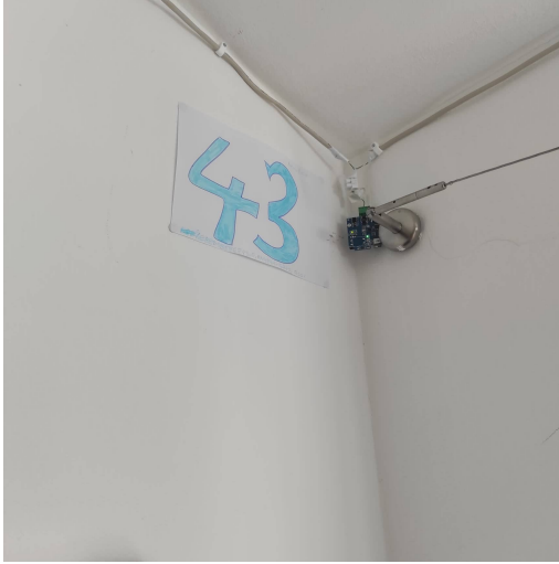
Figure 5.5: Installation of beacon 43
