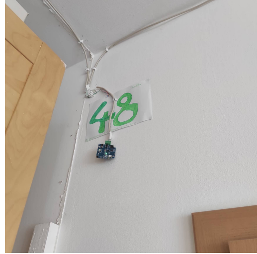
Figure 5.6: Installation of beacon 48
