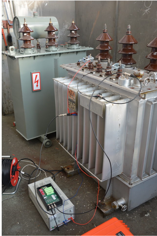
Figure 66. The photograph of the tested transformers. The Object A is in the foreground of the picture.
