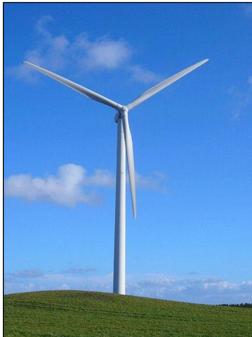
Figure 5.2 – Horizontal axis wind turbine [14]
