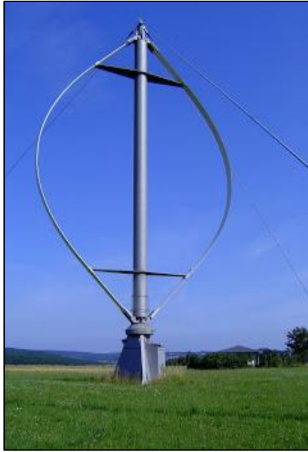
Figure 5.3 – Vertical axis wind turbine [14]
